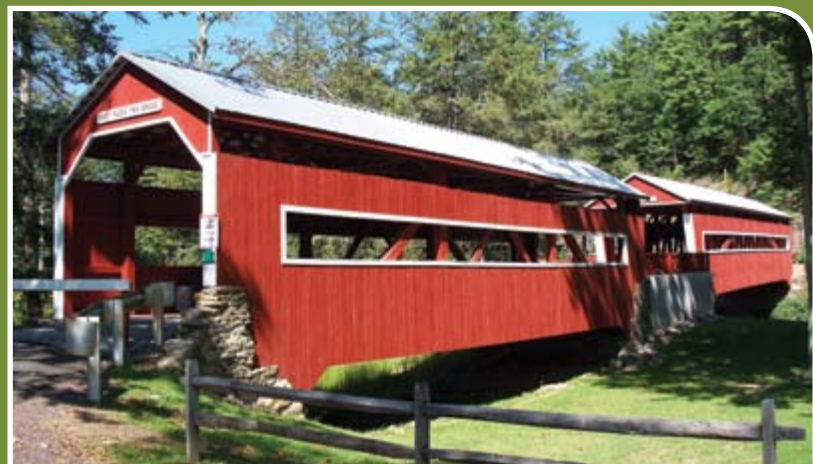
Twin Covered Bridges
