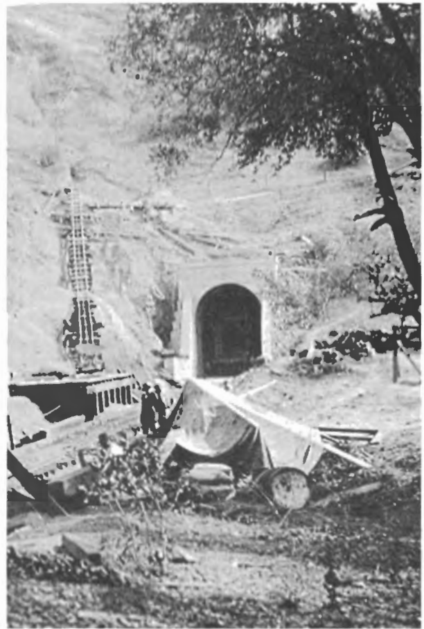
Crews working on the east portal of Tunnel #2 at Summit.
