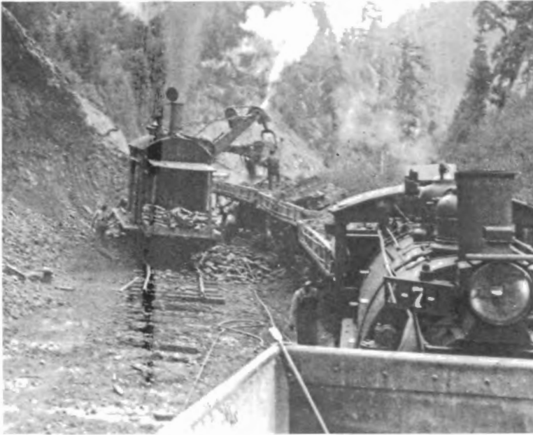
CWR Engine #7 moving a string of side dumps as a shovel makes grade. Engine #7 was a 1909 2-6-2 T, which was re-numbered to CWR #17 in 1924. She was scrapped in 1938.
