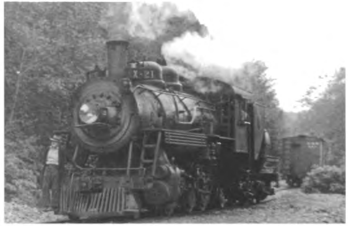
CWR engine #21 working on some light rail. CWR Engines #21, #22, and #23, all 2-6-2s, were built by Baldwin Locomotive Works specifically for the demanding grades and curvature of the California Western RR. Engine #21 still survives in Mexico.
