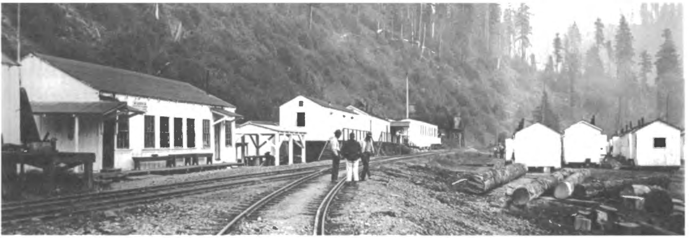
Camp 2 on the CWR's Ten Mile Branch.
