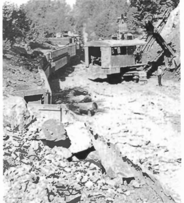
A shovel works the gravel pit at MP 5.7.
