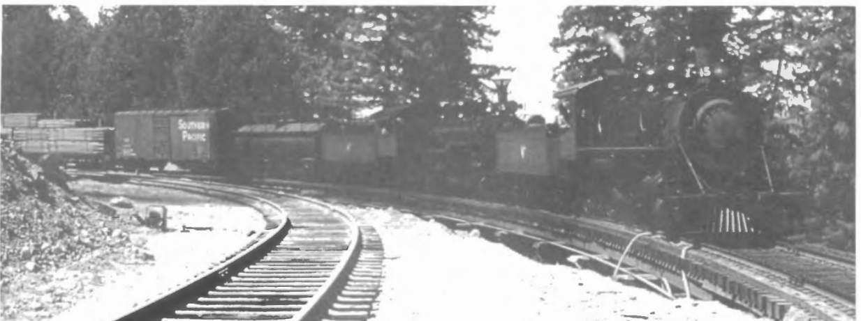
The new track at High Fill, MP 31.3, is nearly complete, but the double-header takes the old trestle as the train moves up the grade toward Crowley. The trestle would soon be abandoned.
