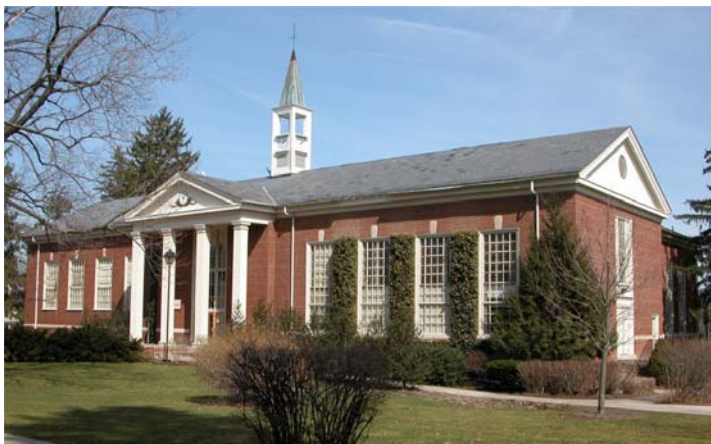
The Blough-Weis Library in 2008, entrance facing West.
